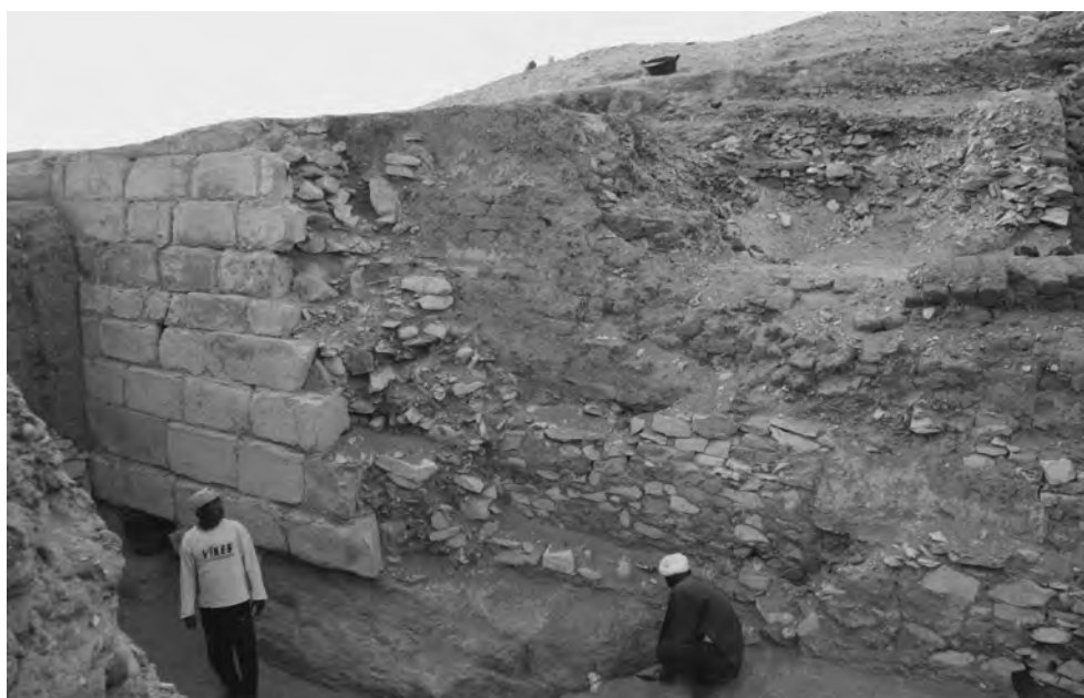
Fig. 3 The northern wall of AS 69 showing its method of construction (photo H. Vymazalová)
